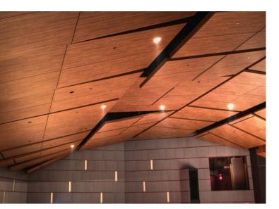
Flat Panel Series 6 (SS6) is a sloped large format ceiling system. Each panel suspends with a hanger brackets from Armstrong® Prelude® XL® Grid or CRS Channel or Unistrut® for suspension.
